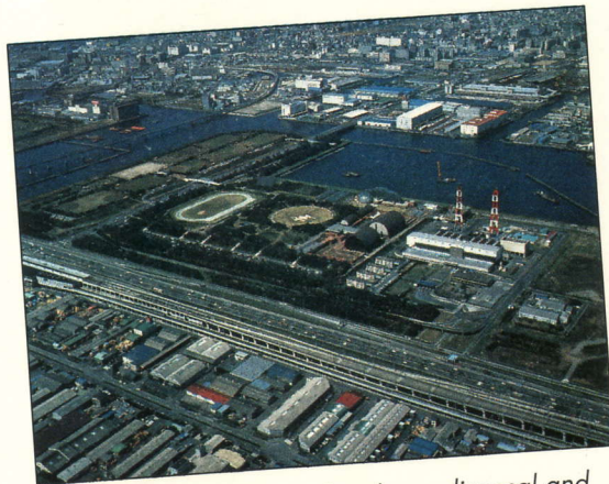
In Tokyo, the problems of garbage disposal and the need for recreational space have been addressed by constructing Dream Island , a containerized landfill island in the harbor.
